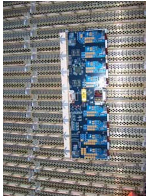
MMR Octapak laying against the array face
