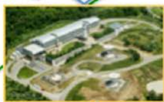
Fairmont Command & Data Acquisition Station
