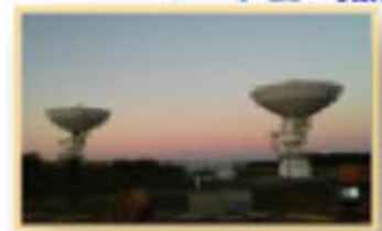
Wallops Command & Data Acquisition Station
