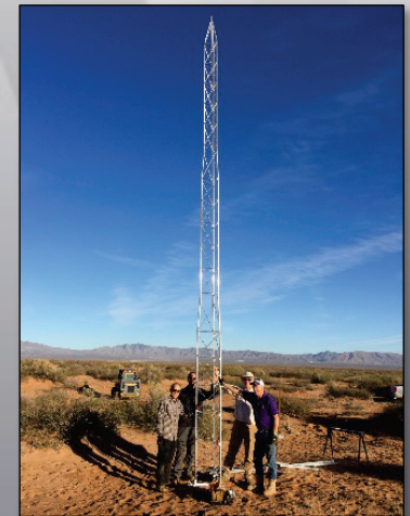
1 st tower installed 1 Dec 2016
